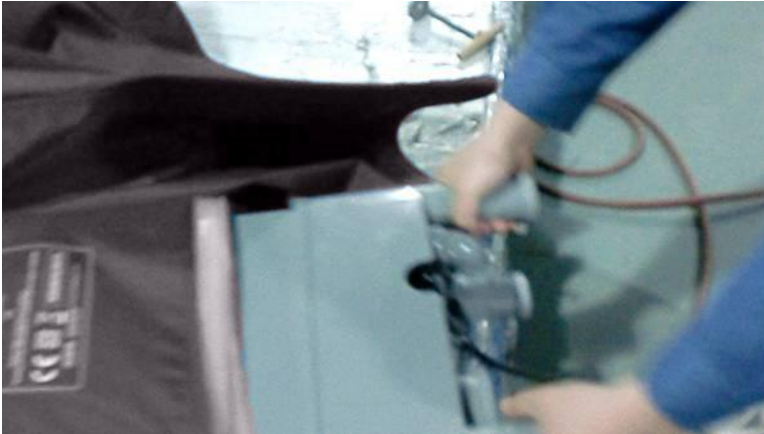
5. Take out control box from spa pool
