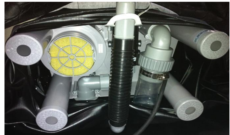
4. Turn the control box inside the spa pool upside down
